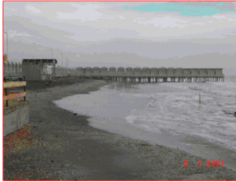
Figure 7 - Section 2: South “Vecchia Pineta” before BMS construction
