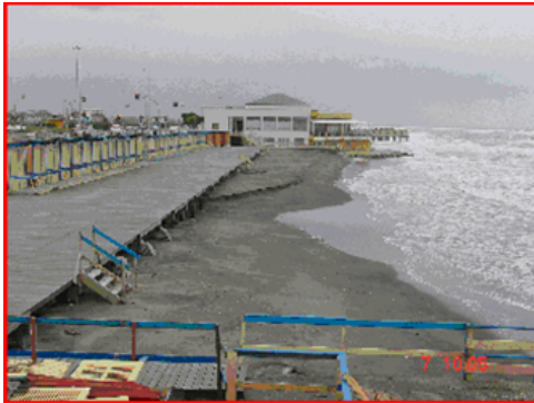
Figure 5 - Section 1: North “Vecchia Pineta” before BMS construction
